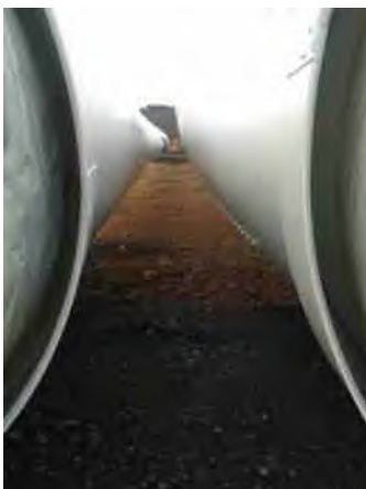
Figure 30: Example of a well prepared area between blade fingers.
