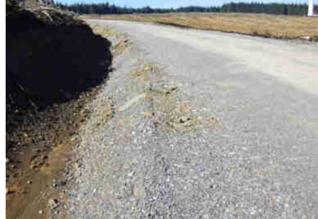
Figure 9: Example of a well-groomed gravel road with a slope for proper drainage.
